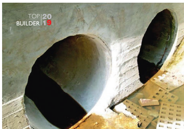
Fot. arch. Aarsleff
